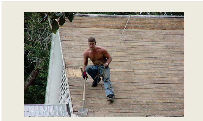
Falls in Construction Re-Roofing
