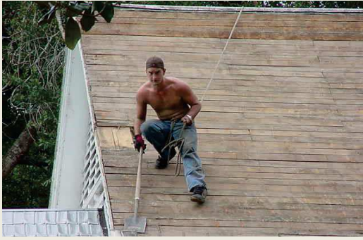
Falls in Construction Re-Roofing http://www.dol.gov/dol/media/webcast/20111031- osha/reroofing_fnl_eng_web.htm
